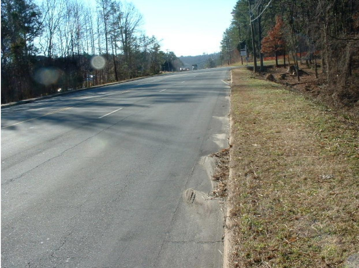
**Image 1.** Clearly visible longitudinal crack in the asphalt covering a concrete 2-foot wide debris-filled gutter pan. MLK Jr. Blvd., Chapel Hill, NC.
